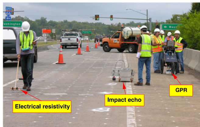
Fig. 1. State-of-the-art of the NDE technology for bridge deck inspection and evaluation.
