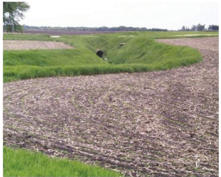
Figure 8: Subsurface drains eventually connect to outlets and ditches that transport cumulative drainage flows to streams and rivers.
