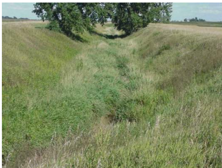
Figure 27: An open drainage ditch in Minnesota (from Needelman et al., 2007).
