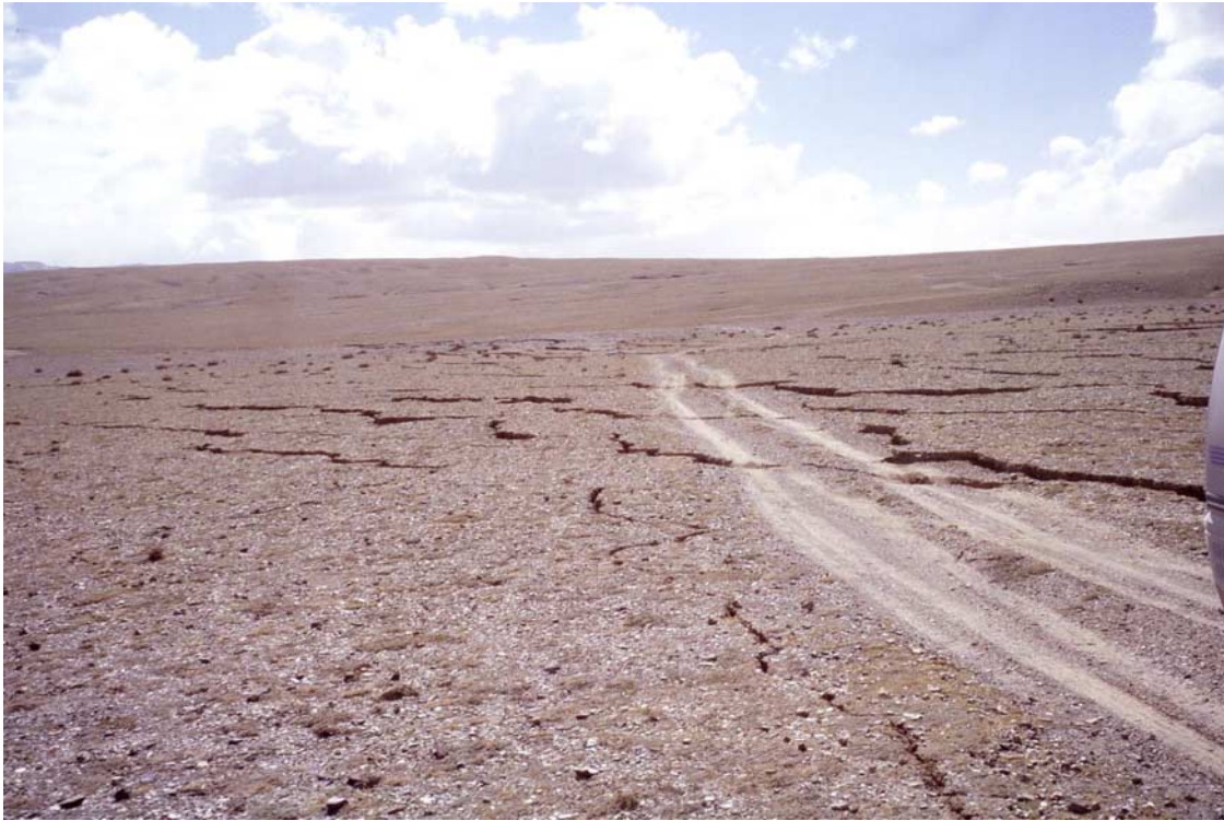
Figure 5. Cracks along the road from Kusai Hai to the Kunlun pass. At this point, the road is several kilometers from the fault. The cracks were not mapped and their orientation was not specifically measured, but was close to the orientation shown in Figure 4. The cracking is consistent either with extension or with compression and inelastic yielding followed by tensile failure when the compression was relaxed.
