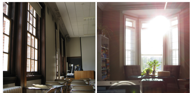
Figure 2: Large, north-facing windows can be effectively used to illuminate spaces such as the classroom shown in the left image. However, glare (when the brightest part of the room is more than seven times brighter than the darkest part of the room) can reduce contrast and visibility. Direct sun far exceeds this range.
