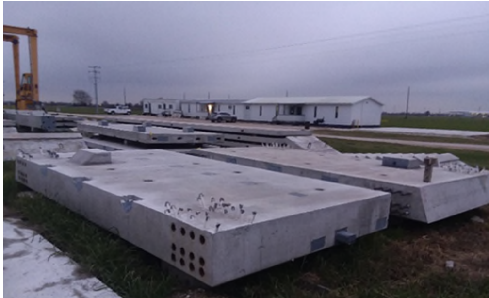
Typical Shear Walls in Storage
