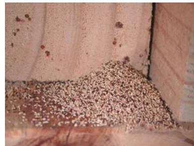
Fig. 5. Drywood termite holes and frass.
