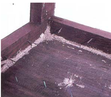
Fig. 6. Subterranean termite mudding.
