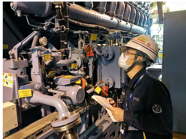
Figure 8. Inspectors Surveying at the Diesel Engine Building of Fuqing NPP
