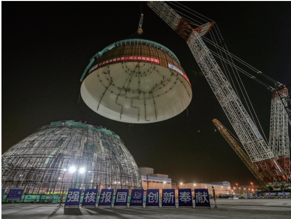
Figure 12. Hoisting and Installation of Inner Dome of Changjiang NPP Unit 3
