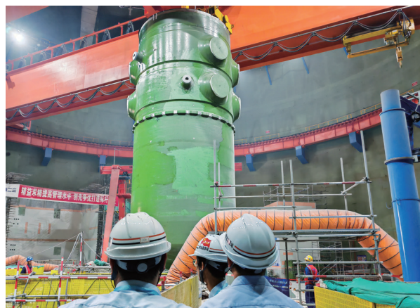
Figure 4. Oversight of Pressure Vessel Hoisting of Tianwan NPP Unit 7
