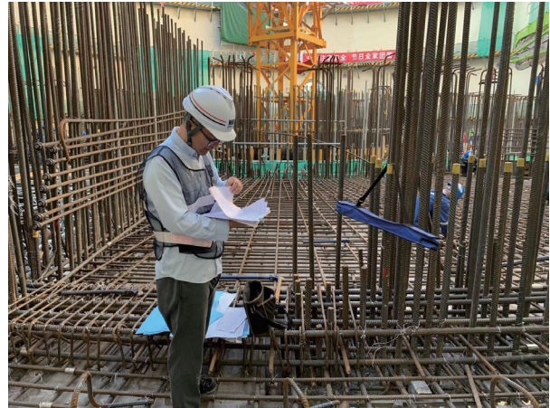
Figure 13. Inspection at Changjiang NPP
