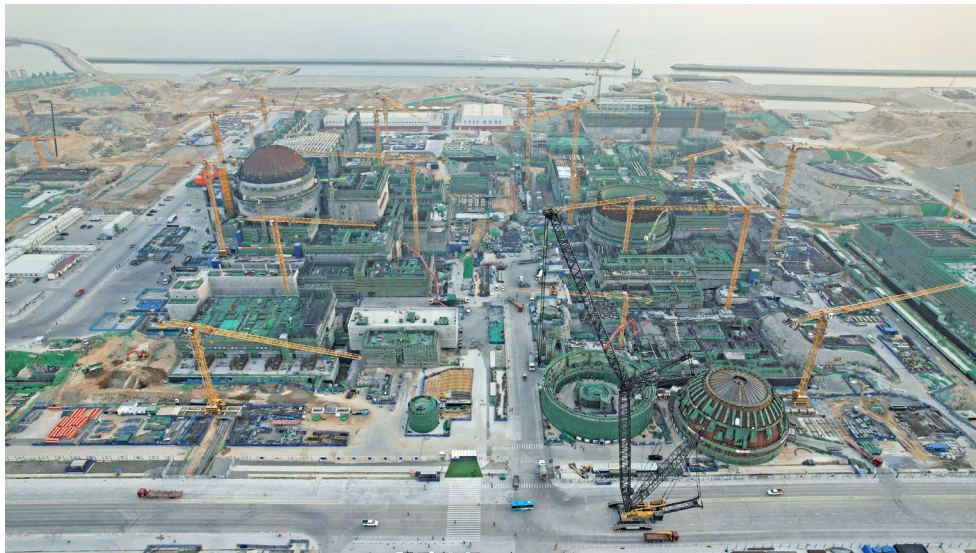
Figure 20. Construction Site of Xudapu NPP Units 3 and 4
