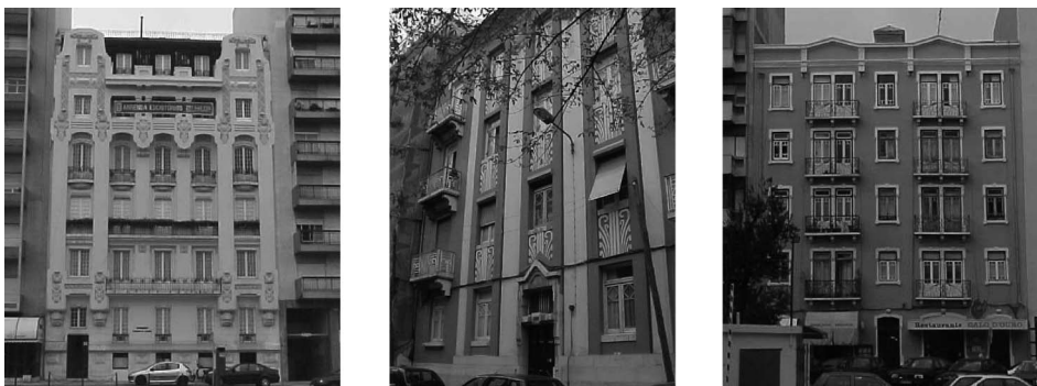
FIGURE 1 Examples of “gaioleiro” buildings, Lisbon, Portugal.
