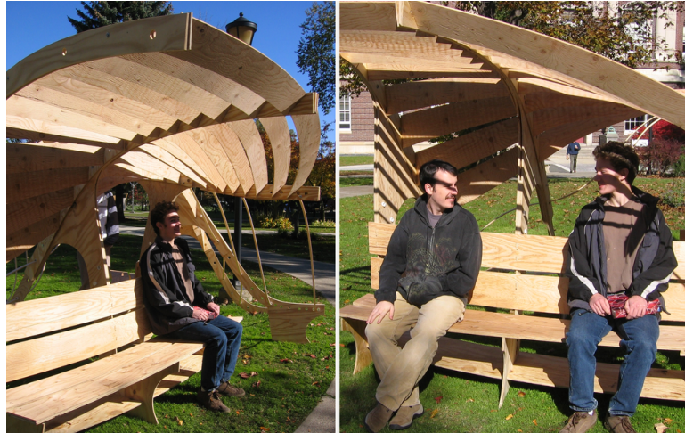
Figure 1.2: Sunlight penetrates the louvres of this architectural studio project in an unanticipated way, causing discomfort. An interactive daylight renderer could have predicted this problem, allowing the designer to optimize the orientation of the louvres.
