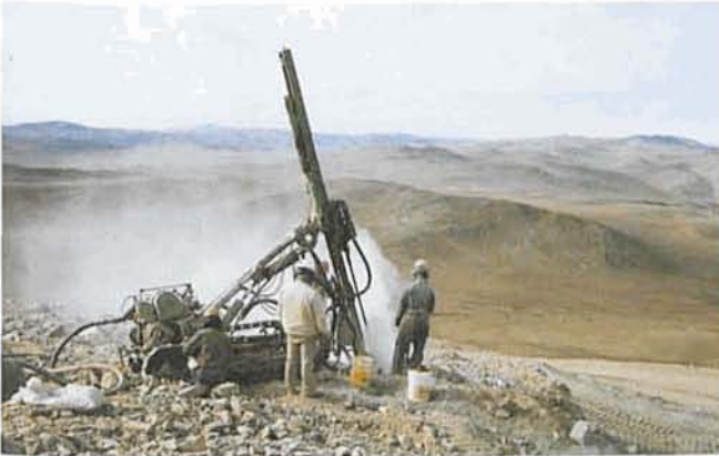
Figure 3: Drilling rig in operation, preparing the next earth removal.
