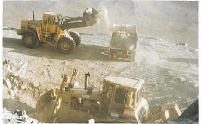
Figure 4: Excavation material loading.
