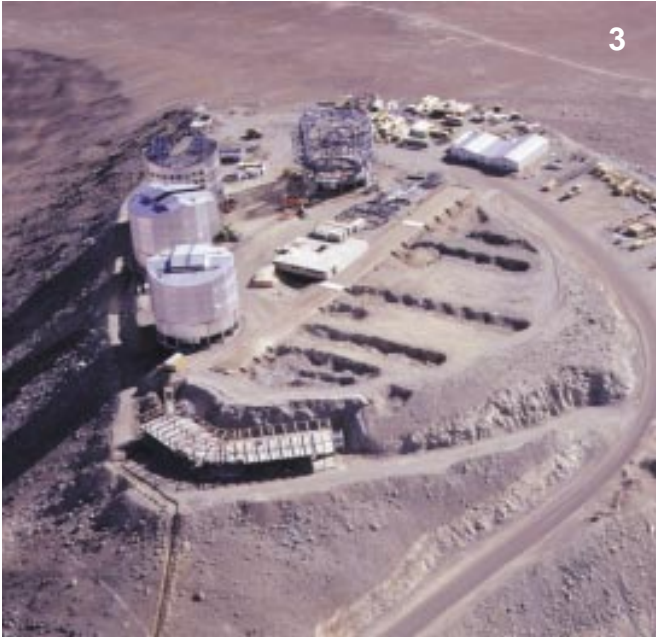
the four enclosures and the steel frame of the control building. In addition, it is possible to see the roof of the delay-line tunnel and the laboratory for interferometry located in the middle of the flat summit area.
