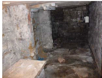
Electricity meter: Barnsley
