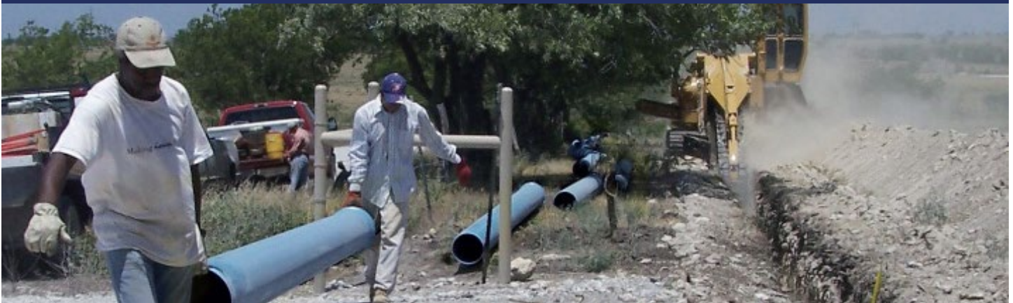
FIGURE 2: MANUAL LIFTING AND PLACEMENT OF PVCO PIPE
