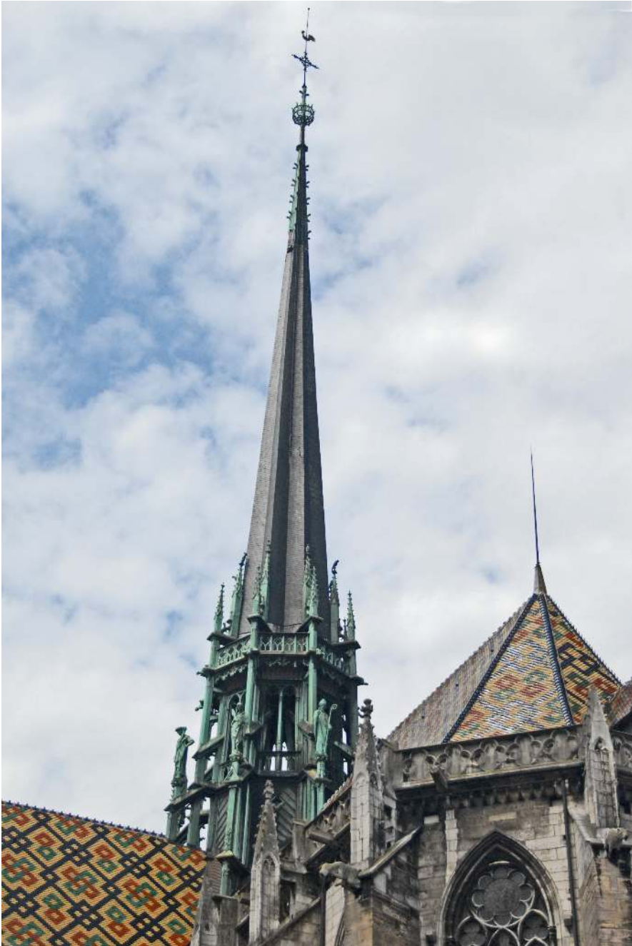
View of the spire of Dijon Cathedral Saint-Bénigne, showing roofs with polychrome tiles. Photo by Jochen Jahnke at German Wikipedia.
