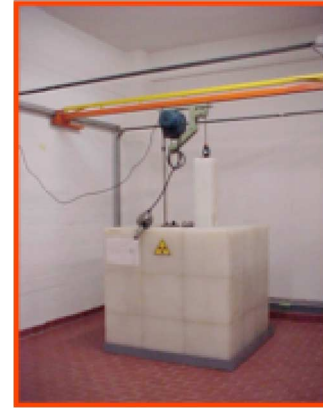
Fig. 2. The thermal neutron irradiation facility.
