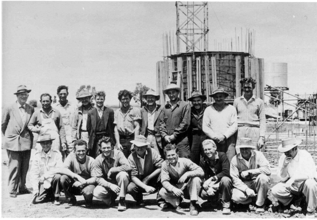
FIG. 11.— The tower was constructed by the Sydney firm Concrete Constructions which recruited most of the tradesmen from the Parkes district.
