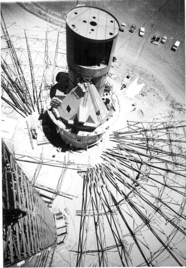
FIG. 12.— (Left) The rib sections of the dish were fabricated on site and welded at night to minimise thermal stresses. A thick layer of sand litters the site, used to sandblast the ribs prior to painting. (Right) Each rib section was lifted into place and bolted to the hub.
