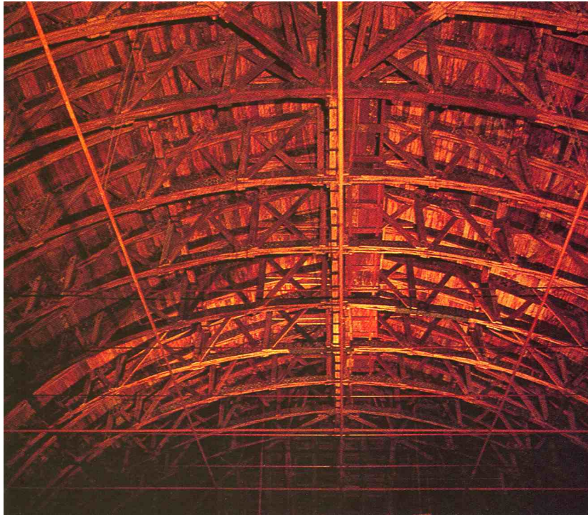
Figure 2. The present wooden vaulted roof of the “Palazzo della Loggia”, Brescia, Italy. (Courtesy of authors of ref. [45])
