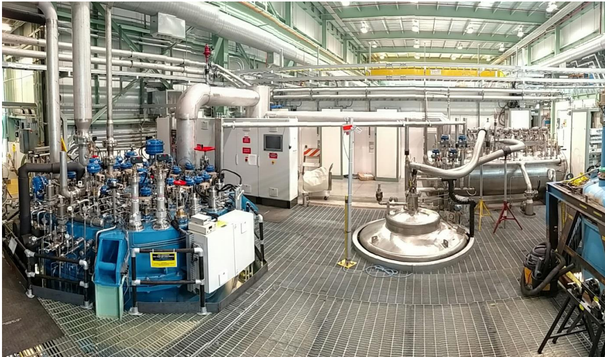
Figure 2: Photograph showing the connections between the SCP, distribution box, and 3000L Dewar
