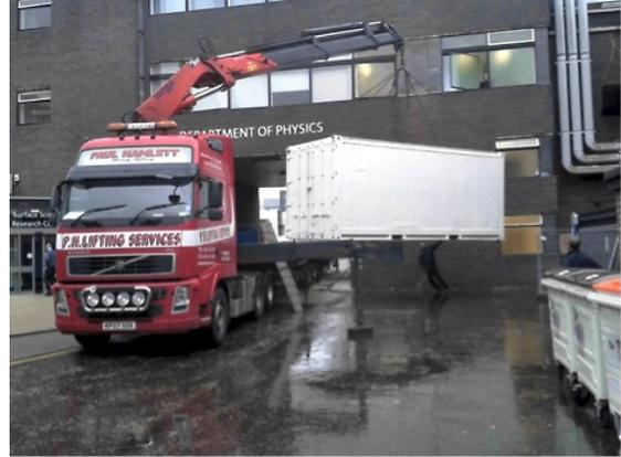
Fig. 24. Loading of the shipping container onto the flat-bed truck, via a HIAB, at the University of Liverpool.
