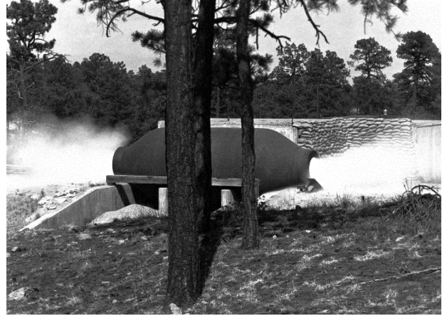
Figure 347. Jumbo #3 in service at Eenie Site, circa 1953. Note the elongated heads, dual manways, and concrete support cradles.
