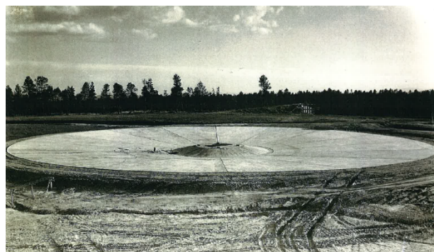
Figure 7. Concrete bowl for recovery of water shots at TA-6, circa late 1944. The bowl is now part of the Manhattan District National Park.
