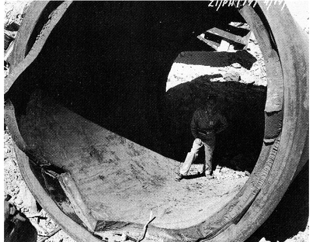
Figure 35. View of the fractured body of Jumbo, April 16, 1946. Note that the vessel did not fail at the welds but in the parent material, providing clear evidence of the welding process quality.
