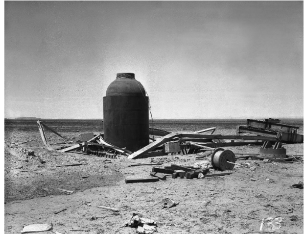
Figure 30. Postshot survey of Jumbo, July, 1945. Note the complete destruction of the heavy-duty erection tower.
