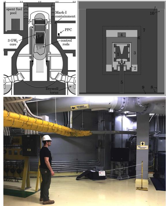
FIG. 1. *Top left:* PPC detector location within the Mark-I design of the Dresden-II boiling water reactor (BWR) [11]. *Top right:* cross section of the detector and shield (see text). *Bottom:* Compact footprint of the assembly, next to the cylindrical primary containment wall. A small cart containing all electronics is visible behind the column, next to the detector.
