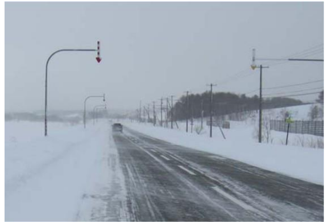
Figure 18: Down-pointing arrow marking the edges of the road covered by snow in Hokkaido, Japan. Image courtesy of Dr. Atsushi Nishimura of Snow and Ice Research Team of CERI (Civil Engineering Research Institute for Cold Region)[247].
