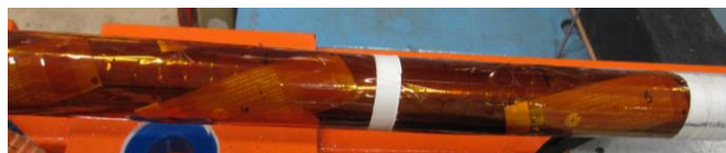
Fig. 2. Flex-QA elements installed on a warm bore tube.
