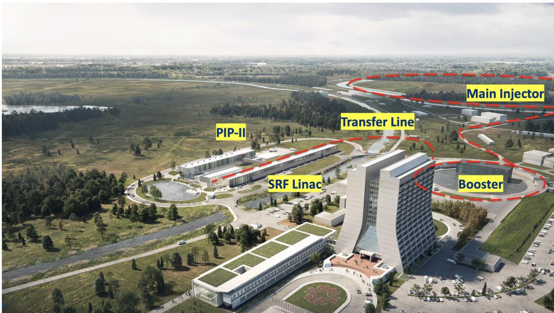
FIG. 1. View of the Fermilab accelerator complex. A rendering of the PIP-II accelerator LINAC is shown in the foreground along with the transfer line to the existing Booster and Main Injector beamlines.
