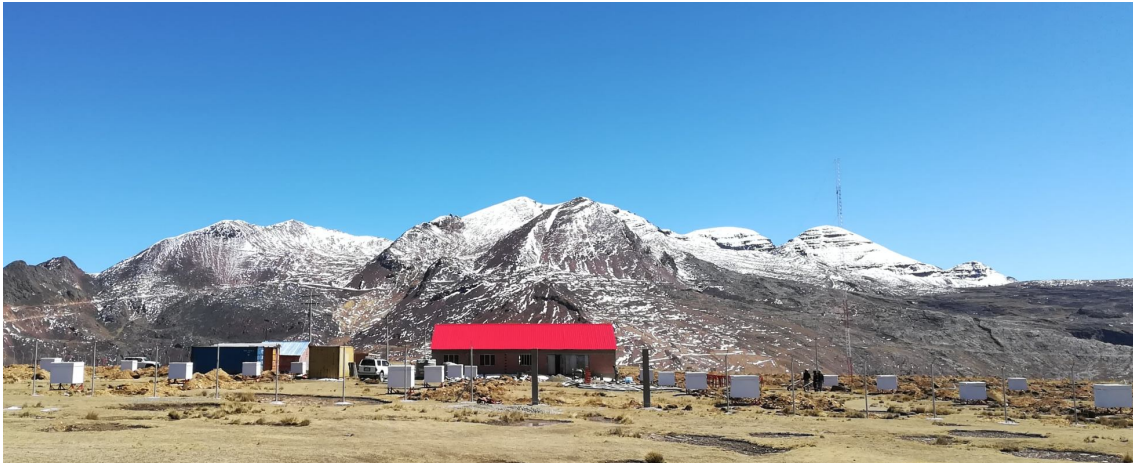
Figure 4: Photo of ALPACA (ALPAQUITA) site. Mt. Chakartaya can be seen in the background. The building with the red roof is the central electronics hut. The multiple white cubes around the hut are SDs.
