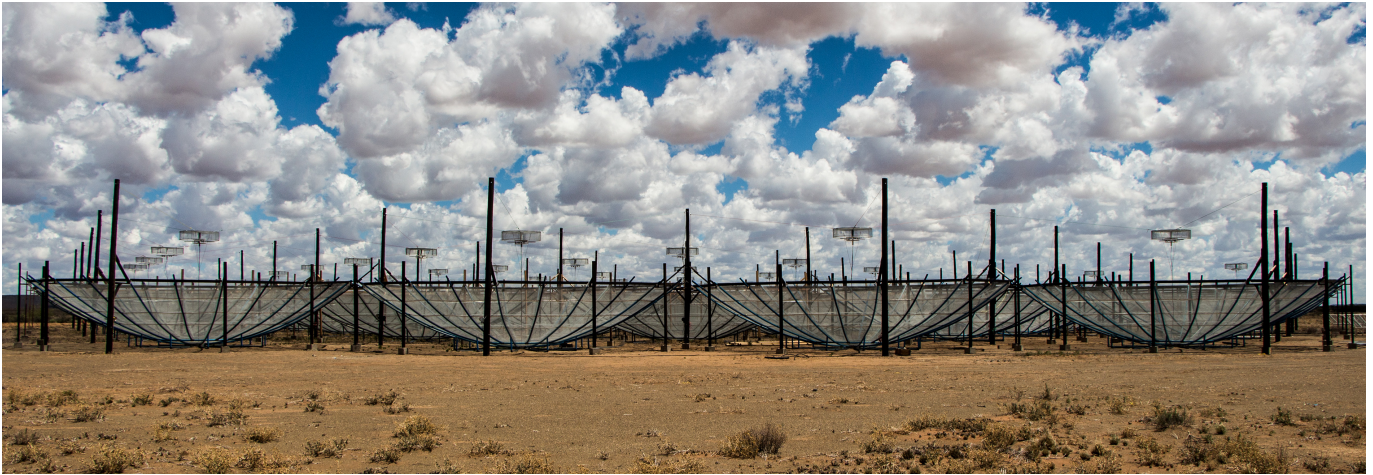
Figure 1. A view of HERA from January 2017. The data in this work were taken during Phase I, when HERA was composed of 14 m parabolic dishes with sleeved dipole feeds in mesh cages suspended at prime focus. These feeds were later replaced with wide-band Vivaldi feeds, expanding HERA’s bandwidth from 100–200 MHz (Phase I) to 50–250 MHz (Phase II).
