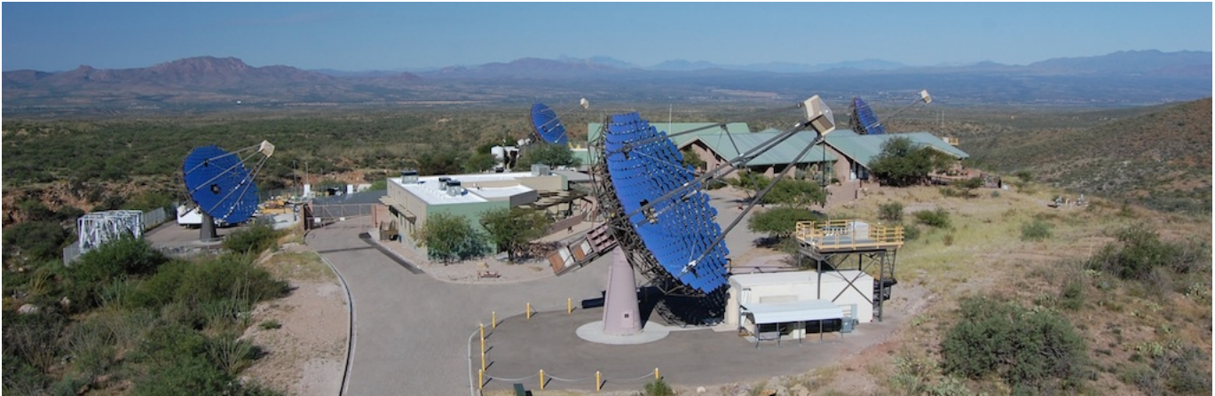
Figure 1. An elevated view of the VERITAS array located at the base of Mount Hopkins near Tucson, AZ. Pictured are the four individual telescopes, which are roughly 100 m apart, the Fred Lawrence Whipple Observatory visitor center, and the VERITAS control building (with the white roof). Image from Abeysekara et al. (2016)
