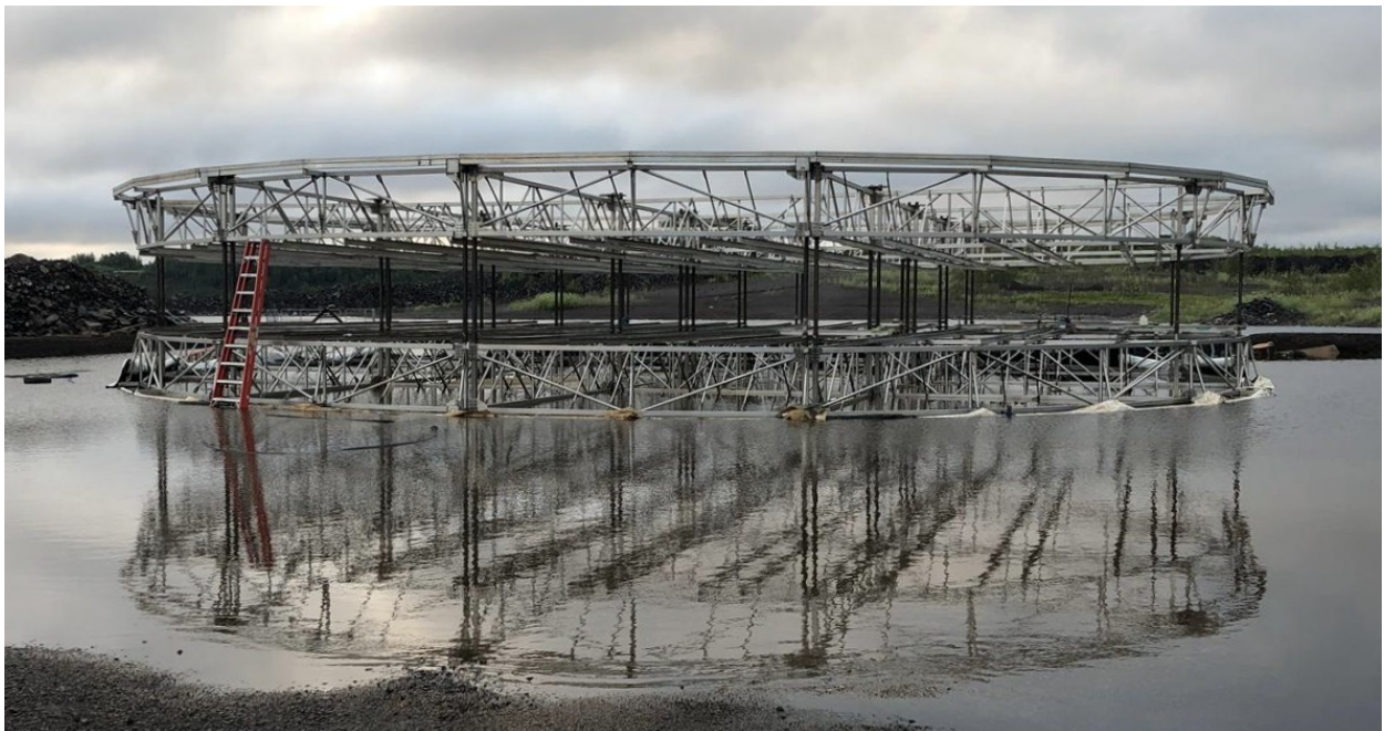
Figure 6: Completed frame. The pillars supporting the top cap are clearly visible.
