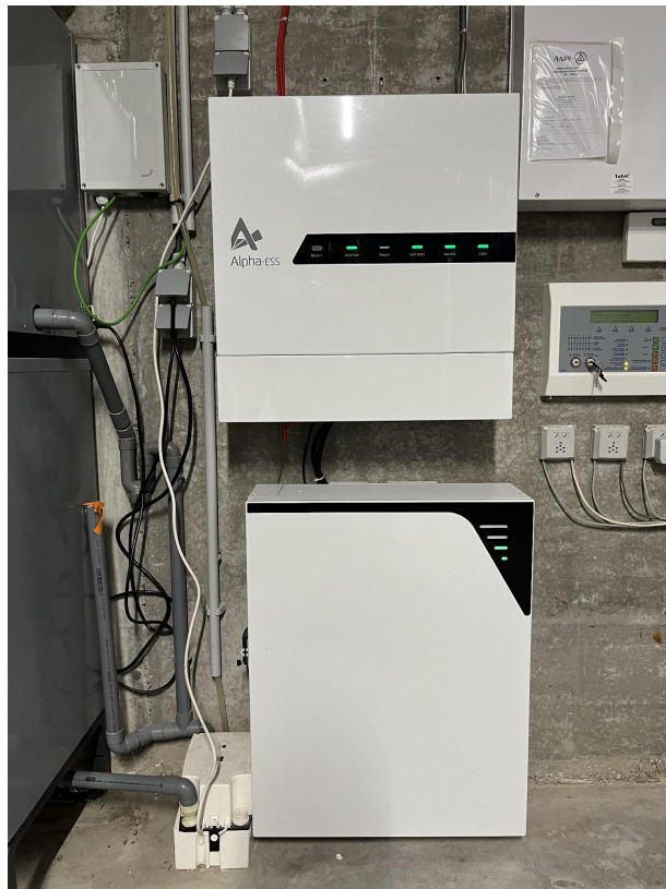
Figure 6: HomeLab battery used for testing the proposed control framework in real world
