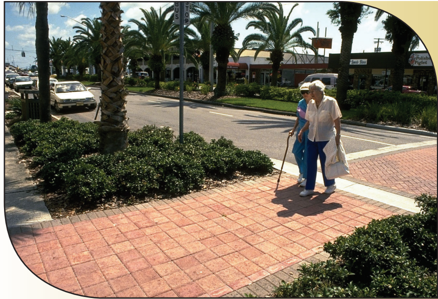
Crosswalk in Venice, Florida. Although attractive, the use of brick or pavers in crosswalks requires regular maintenance to maintain a smooth surface.
