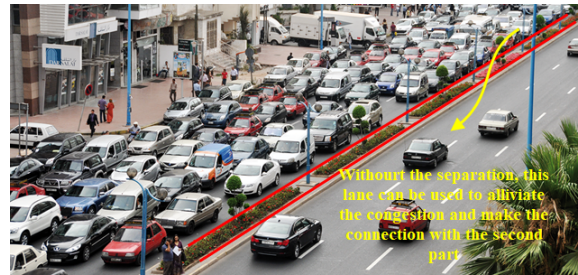
Figure 10: Road with separation between opposite lanes - Morocco
