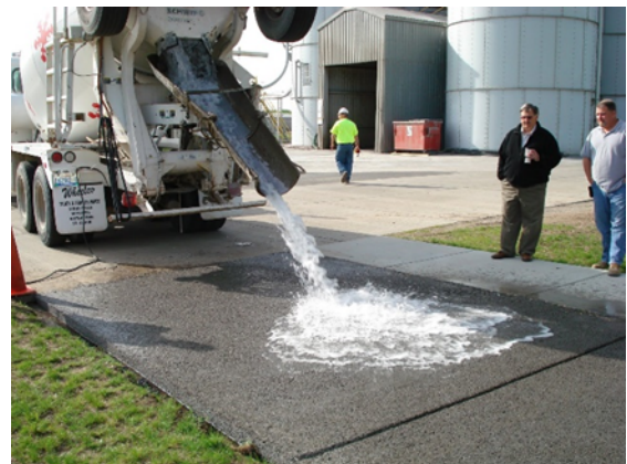
Figure 2: Pervious Concrete Pavement Drain ability (Source: Quick Mix Website)
