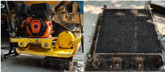
Figure 8: Compaction process for forming APB
