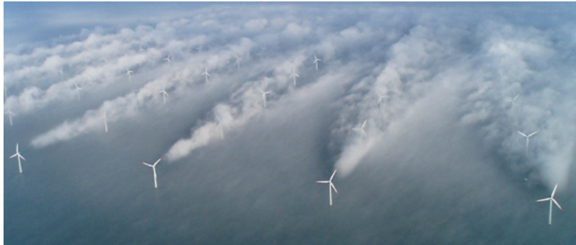
Figure 1: Wake effect on Horns Rev 1 wind park. Many offshore wind parks operating today are still on a regular grid, and so largely affected by wake effect. Source: [21]
