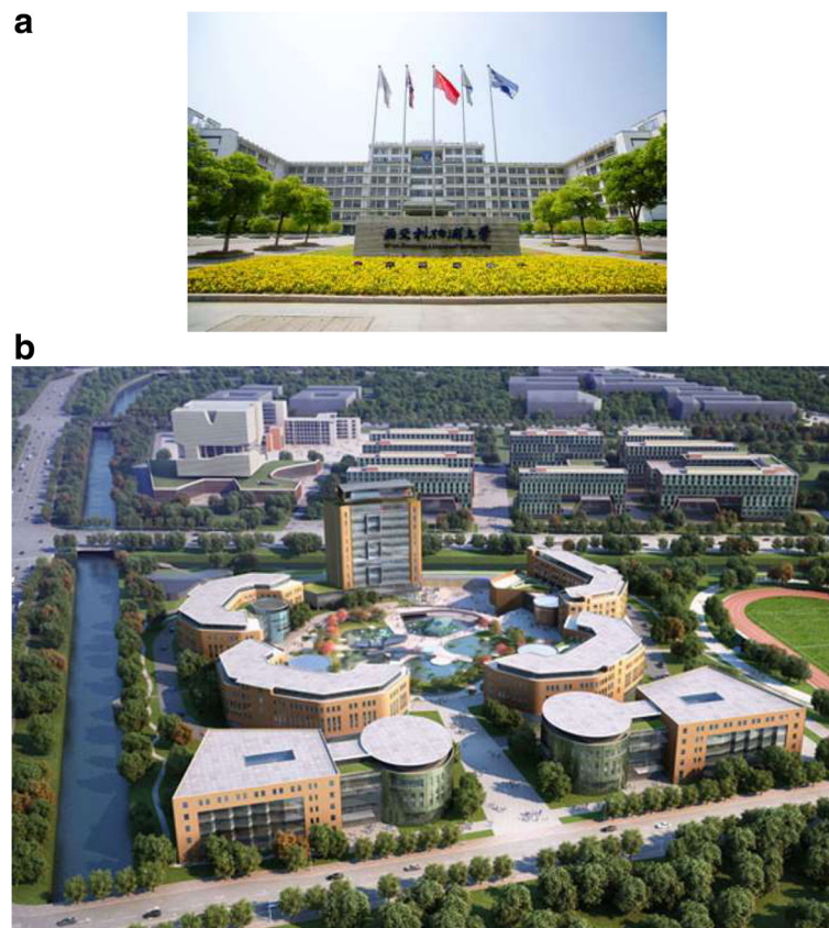
Fig. 3 XJTLU campus in (a) 2006 and (b) 2017
