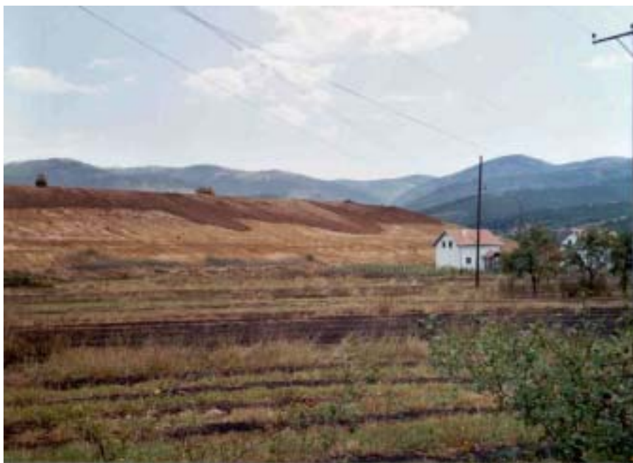
Covering of the perimeter of the tailings area in Gracanica, August 2004.
