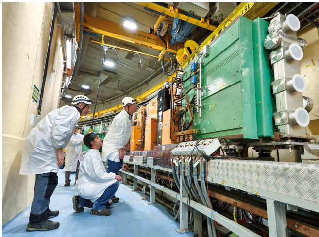
One of the PS Booster's main magnets is dismantled and removed from the accelerator. (CERN-PHOTO-201901-019-1)
