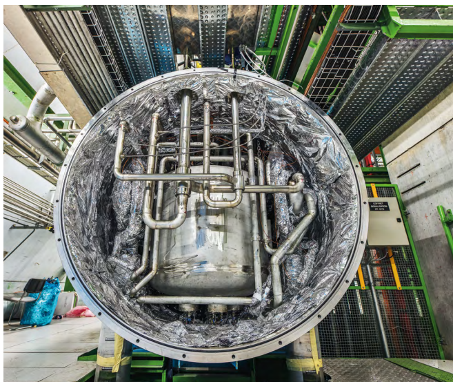
One of the LHC's cold boxes, a key component of the accelerator's cryogenics system, on which numerous maintenance and upgrade operations have been performed. (CERN-PHOTO-201904-107-2)
