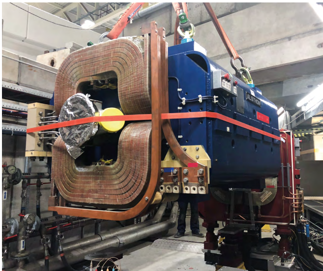
One of the Antiproton Decelerator's dipole magnets is extracted for renovation. (CERN-HOMEWEB-PHO-2020-044-1)
