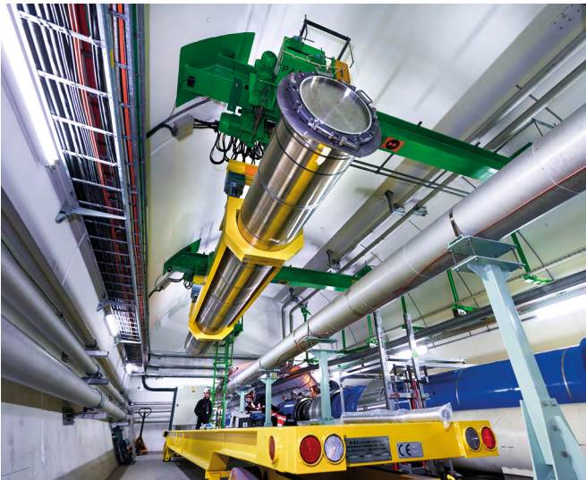
One of the LHC's spare external absorbers is extracted from the tunnel to undergo upgrades in preparation for Run 3 of the accelerator. (CERN-PHOTO-202001-018-15)
