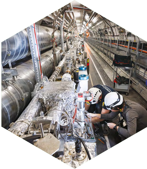
Installation of a new crystal collimator in the LHC for in situ tests during lead ion running. (CERN-PHOTO-202302-036-4)
