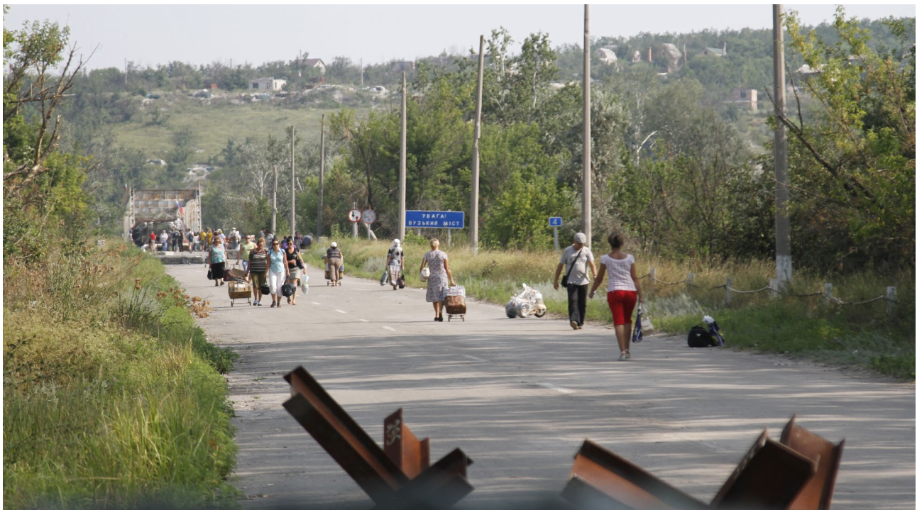
EECP Stanitsa Luhanska, the road to the bridge, the repair of which is blocked by representatives of the ORDLO
