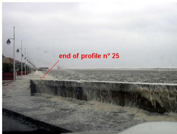
Fig. 5. Submersion of the waterfront walk-way in Leucate-Plage, October 11, 2010. The top of the wall is 2.5 m NGF, its base on the road side is 1.7 m.
