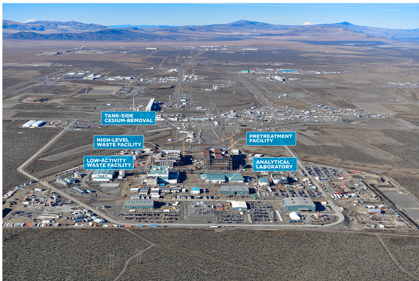
Fig. 4. Aerial photograph of WTP facing west taken in 2020 (snowcaps of Mt. Rainier and Mt. Adams in the distance).
