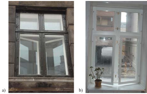
Fig. 4. Energy retrofitted 4-lite of type Window 2 with a secondary frame seen a) exterior of building and b) interior
