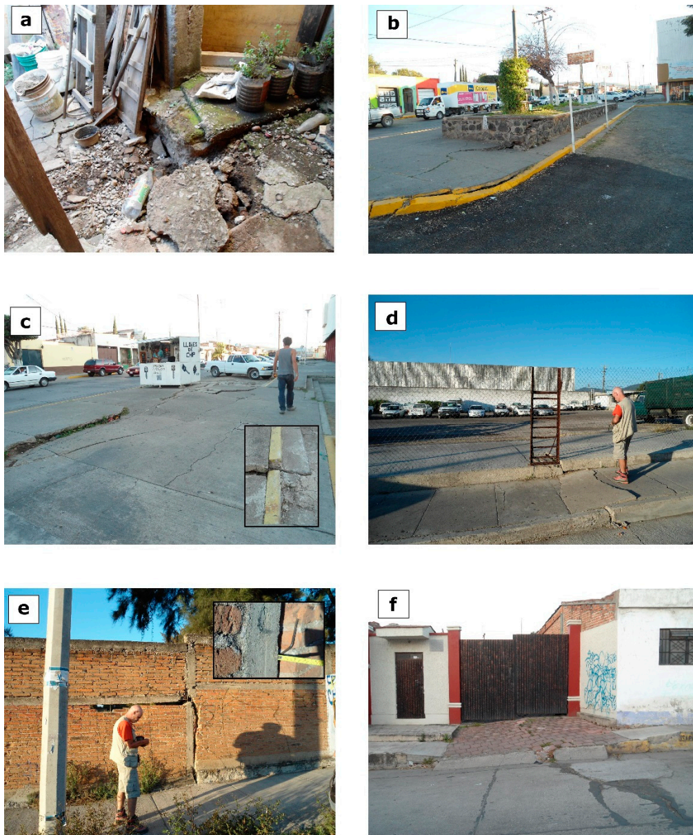
Figure 4. Photos showing evidences of ground fissures and faulting: (a) deformed and fractured pavement (site 1); (b) crossroads and sidewalk showing the pavement displaced and partially repaired (sites 3 and 4); (c) sidewalk affected by normal fault with a minor strike slip offset, as visible in the inset (site 5); (d) parking affected by fissures and normal faults (site 6); (e) sidewalk and wall affected by normal fault associated with a strike slip offset, as visible in the inset (site 10); and (f) street, sidewalk and gate affected by normal displacement (site 11). For the location, see Figure 3.
