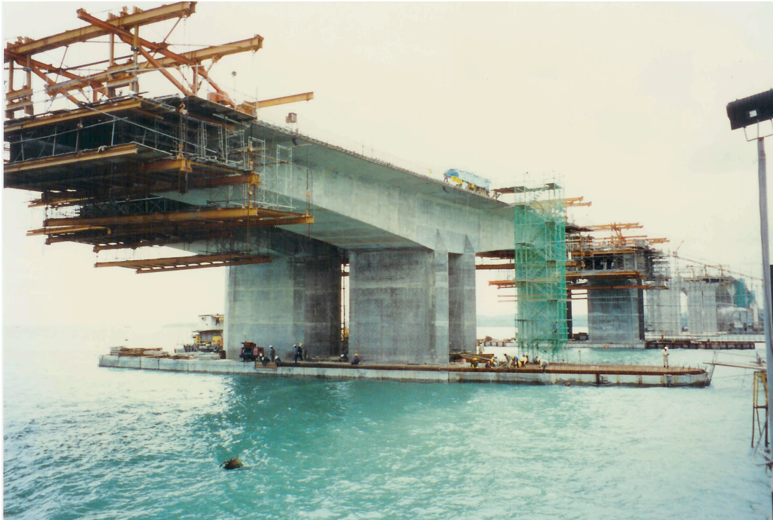
Figure 3 Tuas Second Link under construction, with instrumented segment nearest
