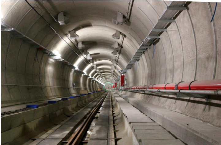
FIG. 7. Measurement conditions during the integrated monitoring with constructed rail bed and fire protective layer on the tunnel section
