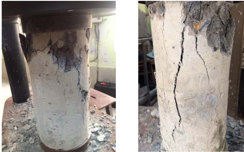
Fig.2 (a) Failure of G4 specimen (b) Failure of GM4 specimen
