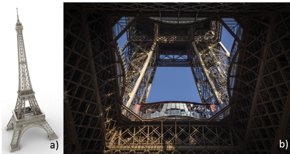
Figure 20 First floor of the Eiffel Tower (Eigensatz, 2012) (a) and (Press) (b): the double-curved facades of the pavilion were geometrically optimized during an integrated design process.
