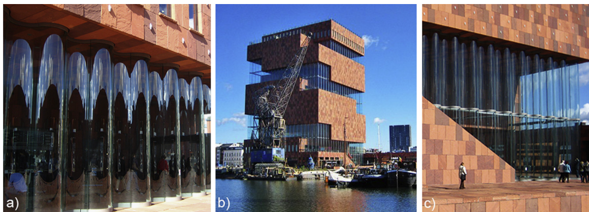
Figure 11 Corrugated panels: corrugated panels can be used as facade (Lisa, 2013) (a-c).
