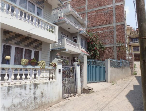
Fig. 28. Settlement and tilting of buildings resulting from ground fissuring.
